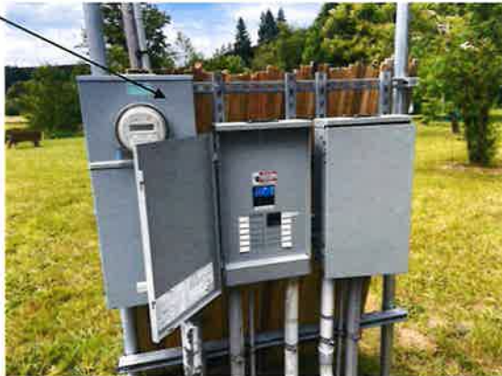
$20k+ electrical work to fix security hazards across the property
